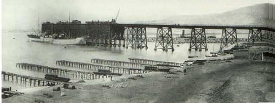
The Alqueje mineral loading bay, also known as the Cable Inglés, a few years after its inauguration in 1904.
