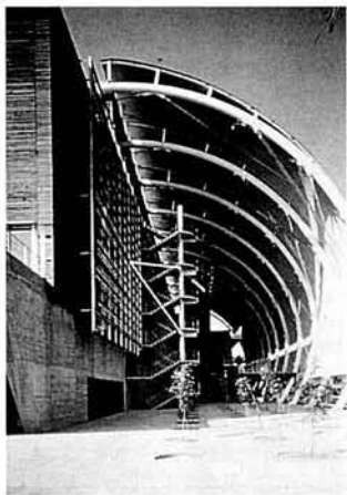
bushhammered concrete was used for the entire building. Inside the floors and acoustic finishes are in wood, and acoustic finishes are in wood.
