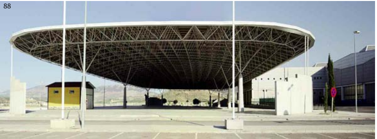
88. Roof over the fair ground. M a Dolores Mateos and Andrés Salmerón, 1999. 89. Former Prados Sanatorium viewed from the accident and emergency building. Manuel Andrades, Jokiñe Uriarte and Armando Vega, 2006.
