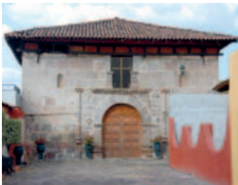
CAPILLA DEL HOSPITAL / HOSPITAL CHAPEL
