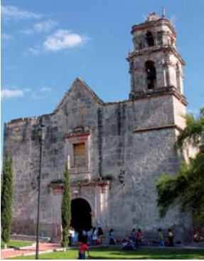
CAPILLA DEL HOSPITAL / HOSPITAL CHAPEL
