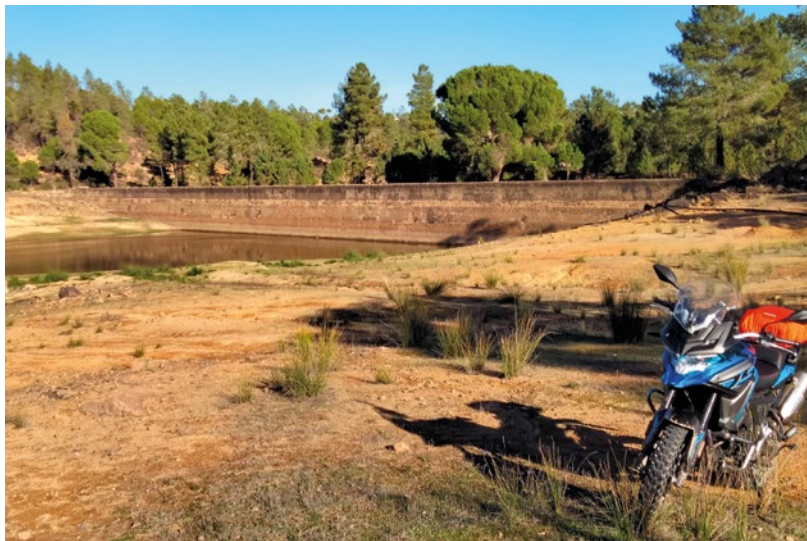
Concepción Mine dam.
