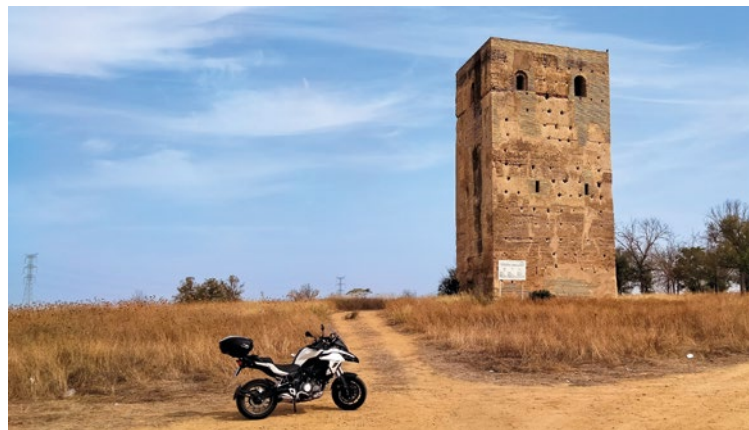
San Antonio tower.
