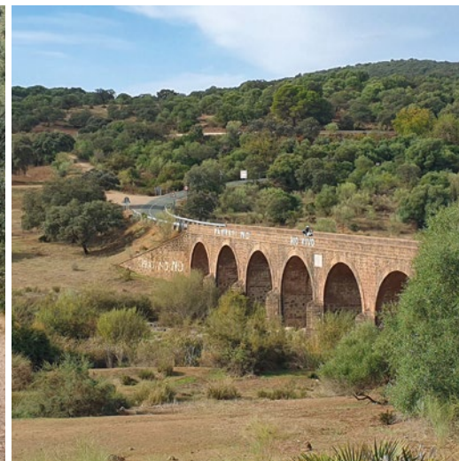
Bridge over River Viar.
