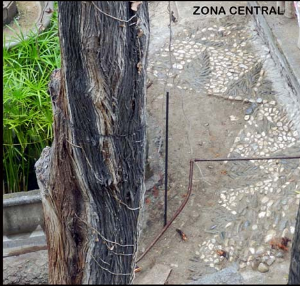
LOSA IN SITU, ZONA CENTRAL
