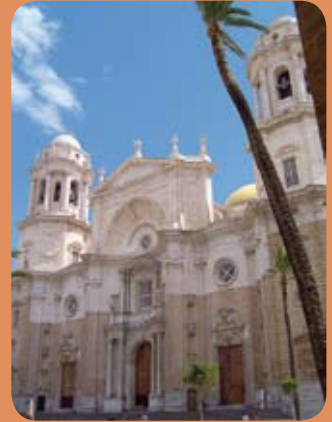
Lower part of Cadiz Cathedral, constructed with oyster stone quarried in the area.
