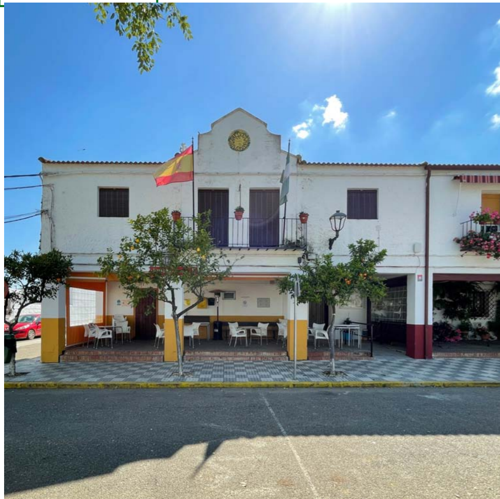
Fachada principal, calle Mayor
