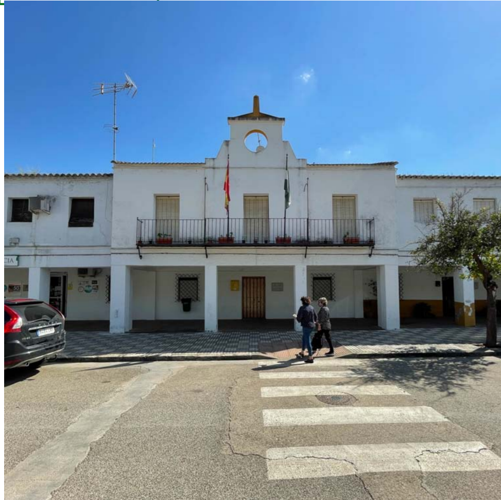
Fachada principal, calle Mayor
