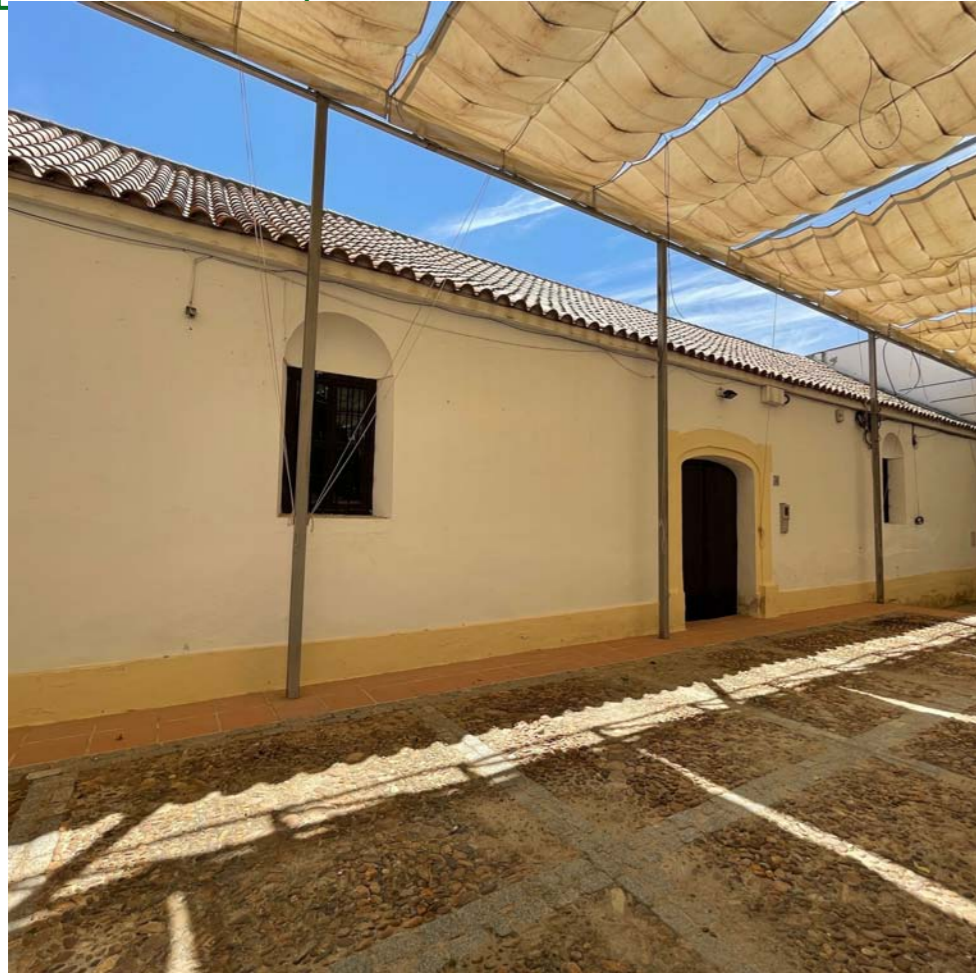
F.Principal patio interior
