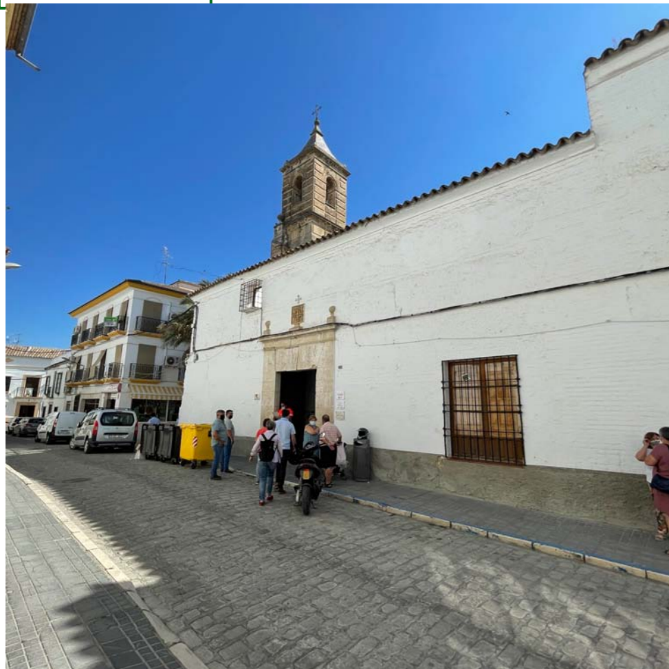
Fachada principal C/ Ancha
