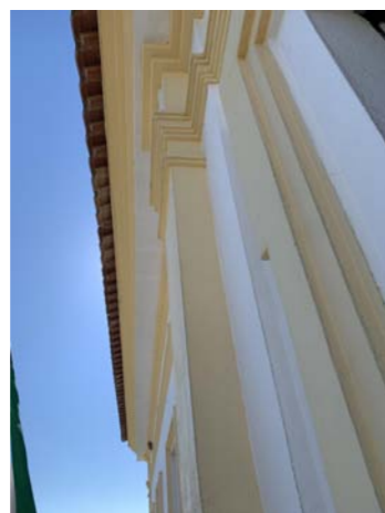
Detalle fachada principal
